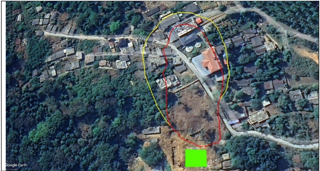
Figure 5.5 Landslide occurred at Govt. Hospital Complex, Upper Gudalur on 17.07.2024
