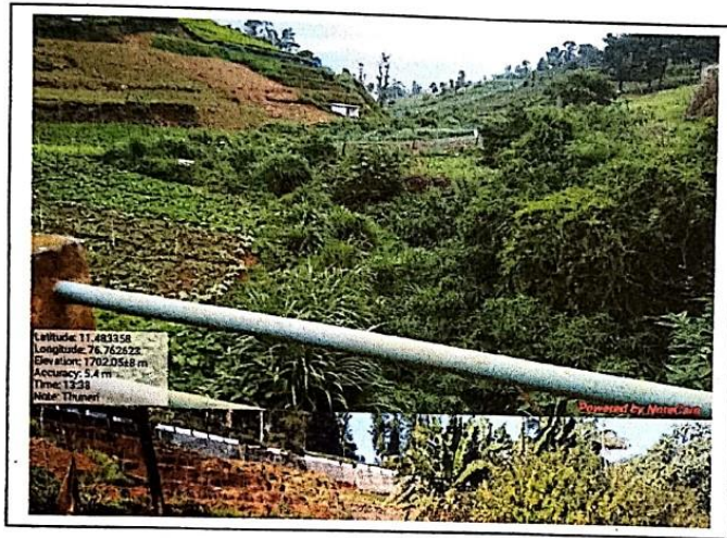
Figure 7.5 - Channel Alignment and Widening works with 1 No. Bed Dam at south side and north side of Thuneri hamlet at a length of 2070 mts and 700 mts in Thuneri Macro in Udhagai Block.
