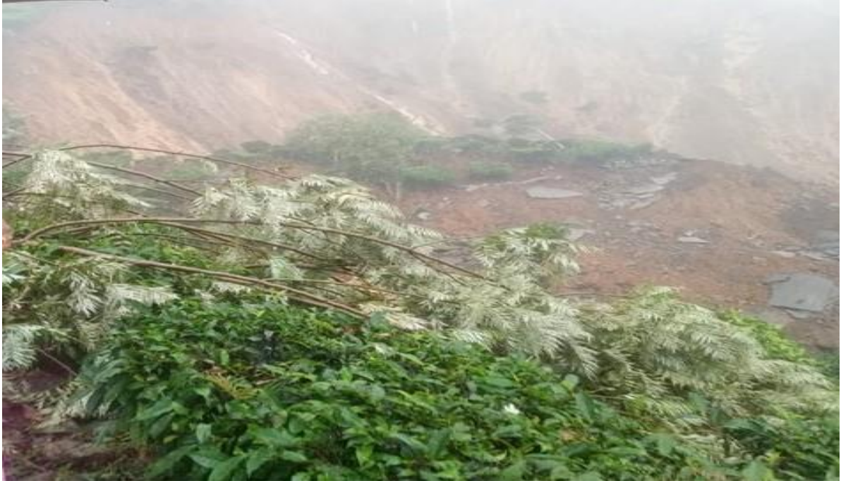
Figure 5.4 - Landslip at Kilkotagiri to Mettukal Tribes hamlet road
