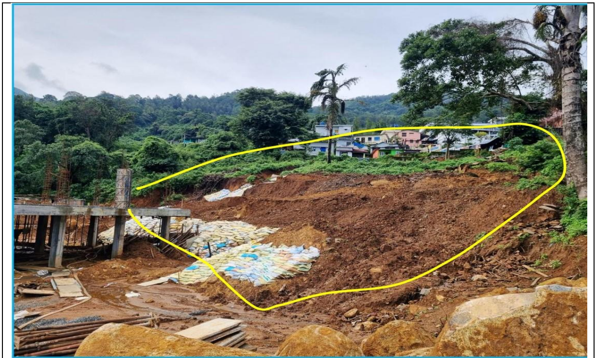
Site specific study has been conducted by GSI at Govt. Hospital, Gudalur 17.07.2024
