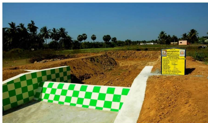
State : Tamilnadu Name of work : Const of Cement Concerete District : Krishnagiri Check dam @ Jeenur Chl.
