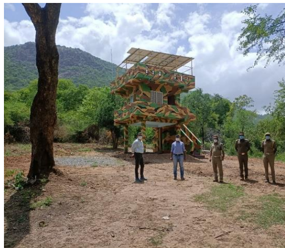
Fig: Watch tower erected with Solar panel @ Tholuvabetta RF, Denkanikottai Range
