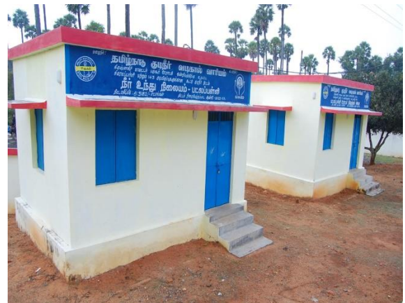
Pump room @ Battalapalli in Bargur union
