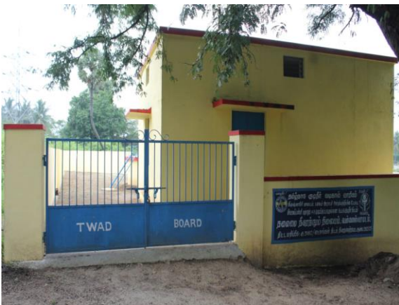
Head works @ Penneshwaramadam in Kaveripattinam union
