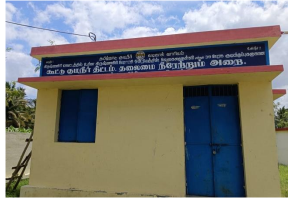
Head works @ Thavalam in Krishnagiri union
