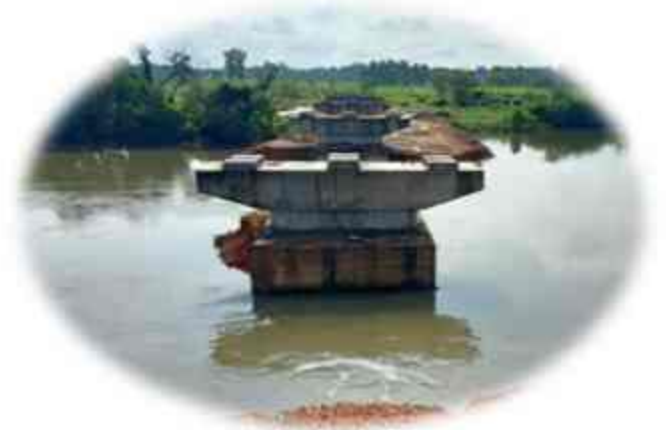
Bridge work in Udupi, Karnataka
