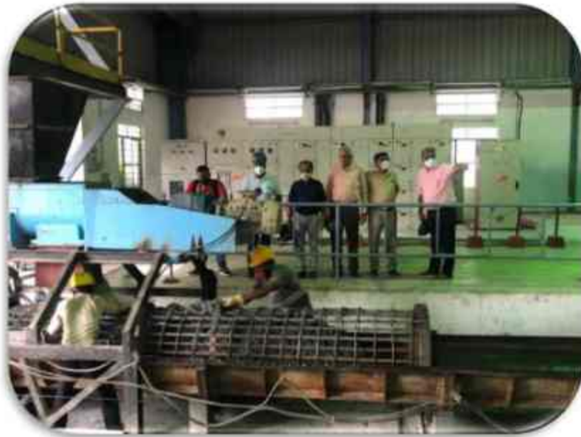
EWDS Spun Tower – Factory Acceptance Test in Goa
