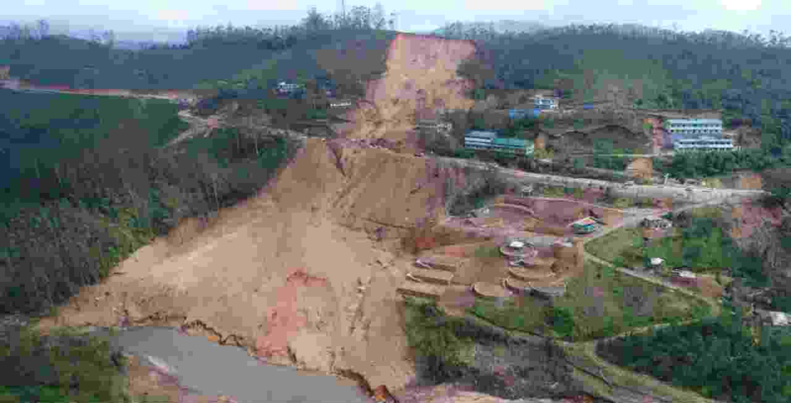
Landslide occurred at Government College, Munnar, Idukki District, Kerala during August 2018
